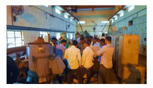
**Observation of Pump Functioning:** During the tour, participants had the chance to closely observe the functioning of the VT pumps. Trainers from KBL elaborated on the different modes of operation, focusing on how these pumps handle varying water levels and flow demands. The trainers provided insights into the mechanical and hydraulic aspects of the
